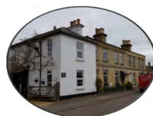
Flat roofed terraces
