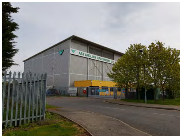
Large factory/industrial unit to the north of Nordic House
