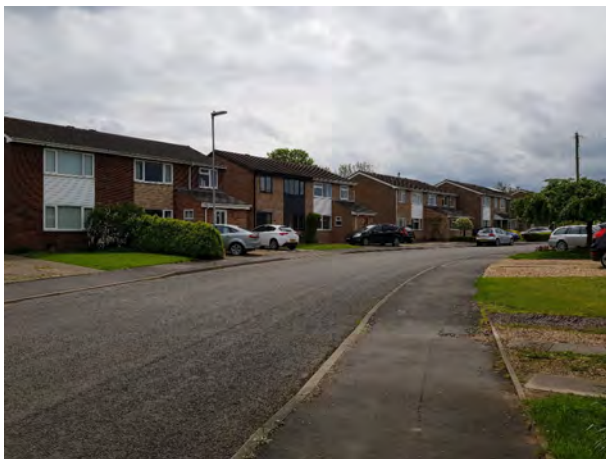
Two storey properties along Headlands with on plot parking
