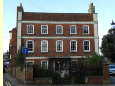
Whitwell House, High Street, Huntingdon
