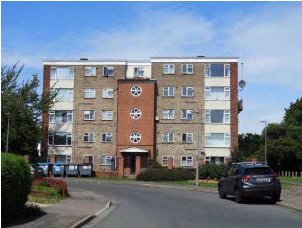
The 5 storey flats provide a focal point on the corner of Duck Lane
