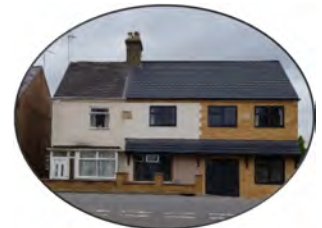
Modern extension to property
