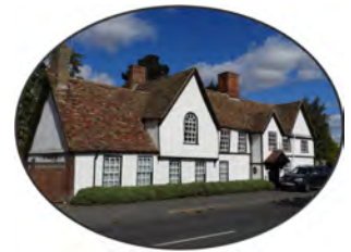
The Old Manor House, 66 Hartford Road
