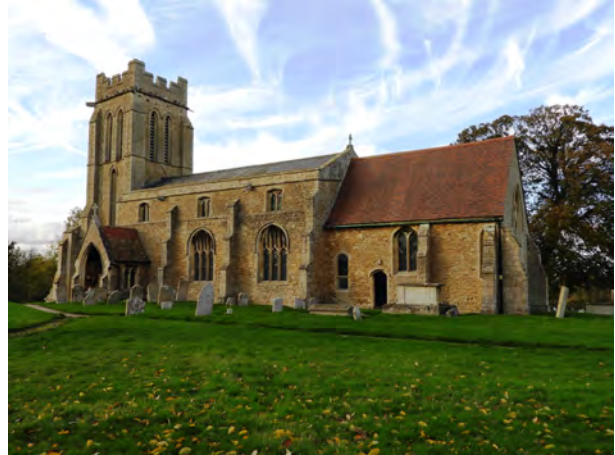
Set high above Warboys Road Holy Cross Church dominates views into this part of the village
