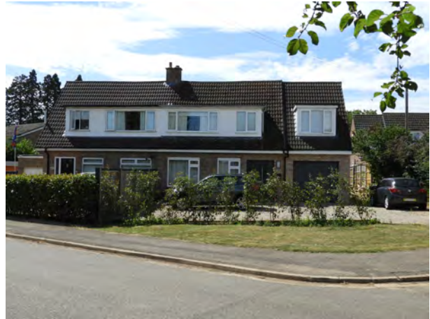
Side extension on a semi-detached chalet style home in Wilkinson Close
