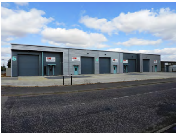
Simple structures in soft grey and neutral shades typify more recent industrial buildings
