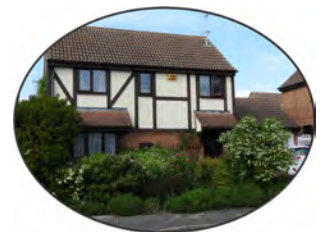
Mock Tudor detailing on Fishers Way
