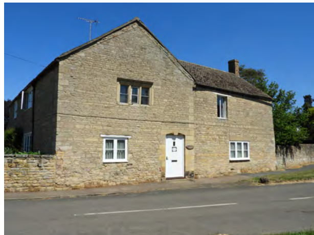
Old Mill House in Elton typifies the use of limestone and Collyweston slates of older buildings in the area
