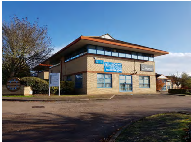
Avro Court business unit demonstrating the architectural detailing and style found within the business park
