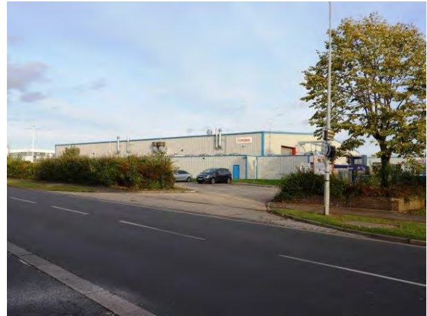
Large industrial unit surrounded by fencing and parking on Cromwell Road
