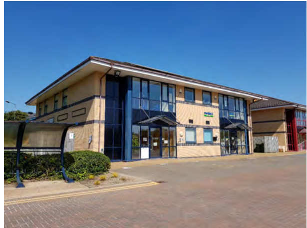
Business unit within Ramsay Court demonstrates colour detailing to add visual interest and cycle parking spaces with some planting
