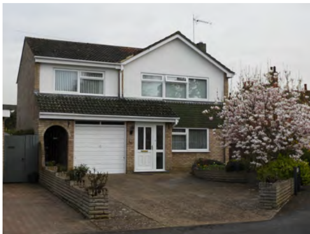
Green hanging tiles and partial rendering provide soft finishes with the detached house set back sufficiently to allow on plot parking
