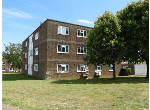
Low rise flats off Duke's Road are set in extensive open space with footpaths linking throughout the local area
