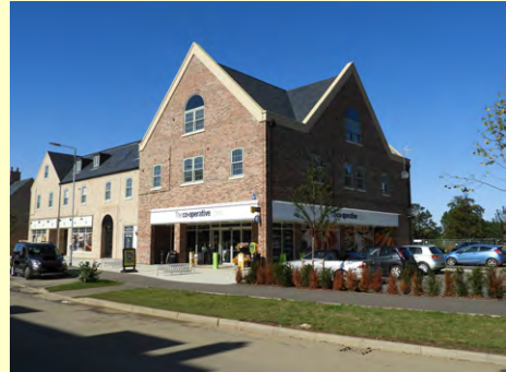
Integrated shop units, Brampton Park
