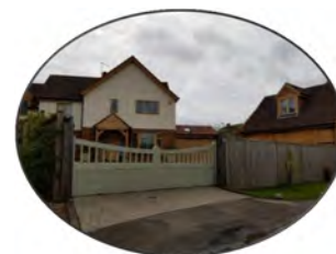
Chapel End modern house
