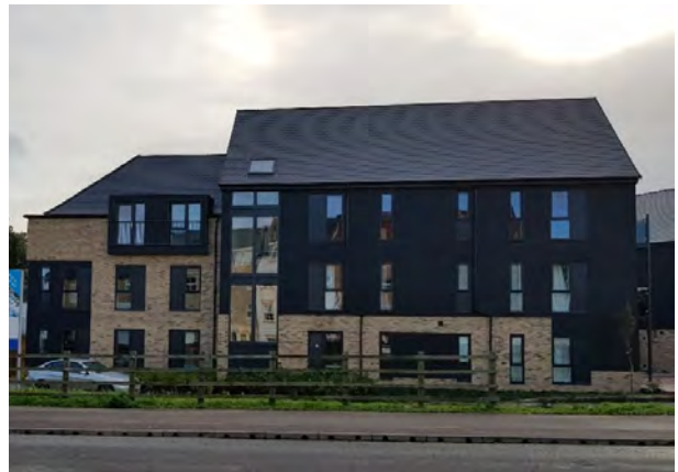
Flatted development on previously developed land, Drovers Place, Huntingdon
