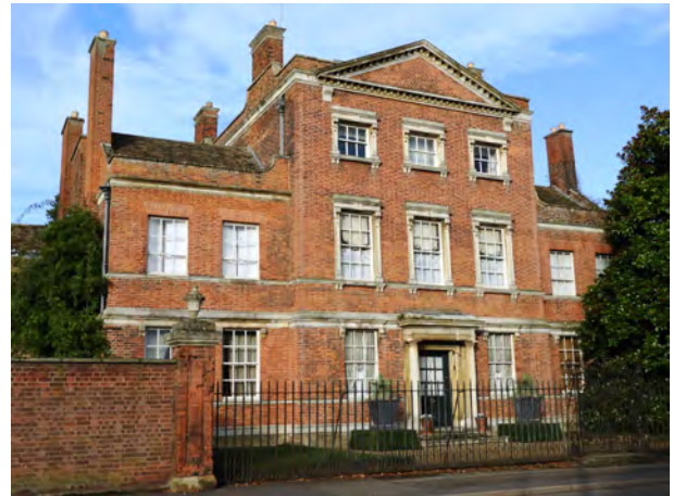
Island Hall faces Post Street opposite Godmanchester Community Academy; it has a symmetrical front of red brick and extensive gardens down to the river including its own island
