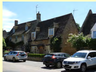
Elton Road, Wansford
