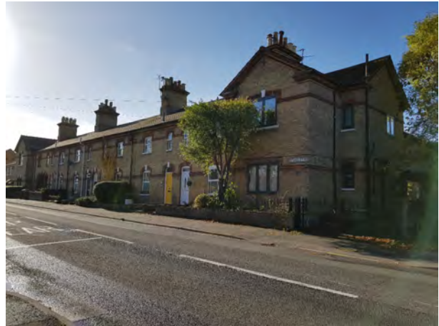
Terraces located along Stukeley Road
