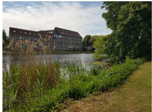
Riverside Mill, a converted Hosiery Mill is located on the banks of the River Ouse next to the historic gateway Town Bridge between Godmanchester and Huntingdon
