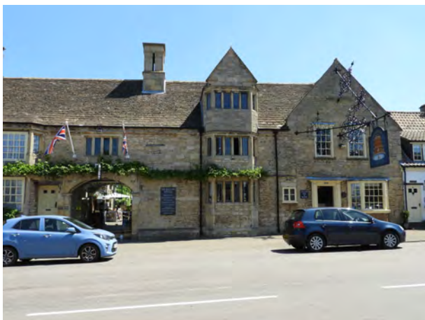
The Bell Inn, Stilton constructed in limestone brings a soft warmth to the streetscape
