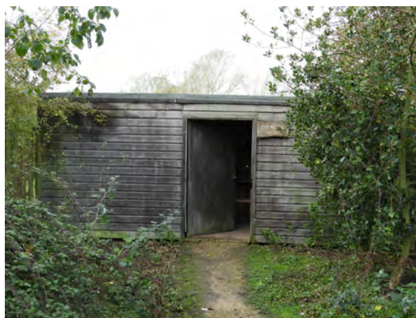
Mander Park bird watching hide provides an opportunity for people to interact with nature without causing disturbance; the wooden building blends well into the surrounding trees and shrubs minimising its impact on wider views
