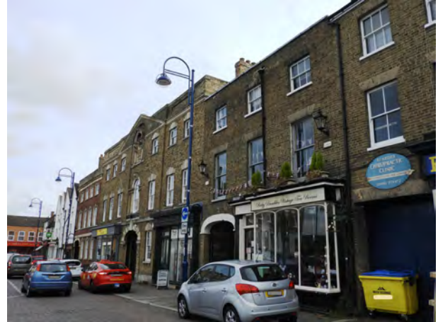
The southern side of the Market Square includes a high proportion of listed buildings reflecting its high townscape value
