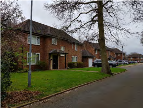
Rectory Close with hipped roofs to property, garages and porches and amenity space
