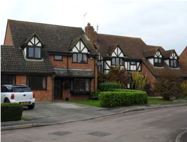
Mock Tudor detailing and brown pantile roofs are prevalent throughout Ashfield
