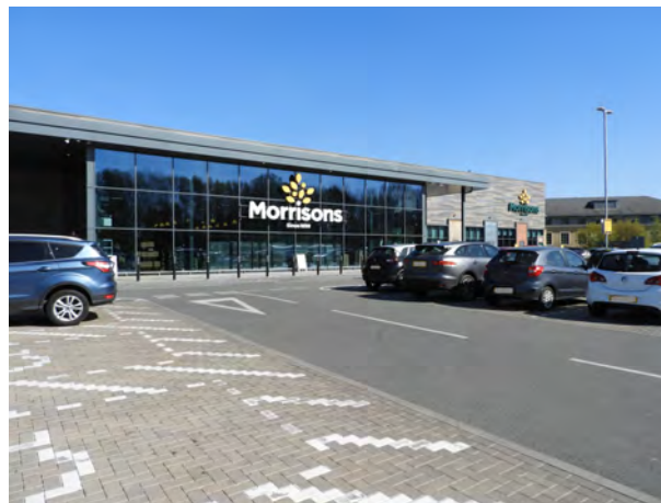
The area offers two large modern supermarkets in simply styled buildings surrounded by surface level car parking
