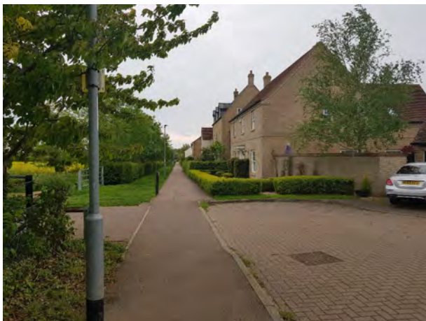
View along Cranesbrook, hedging screens the development from the wider countryside with linkages to the public rights of way and playing fields
