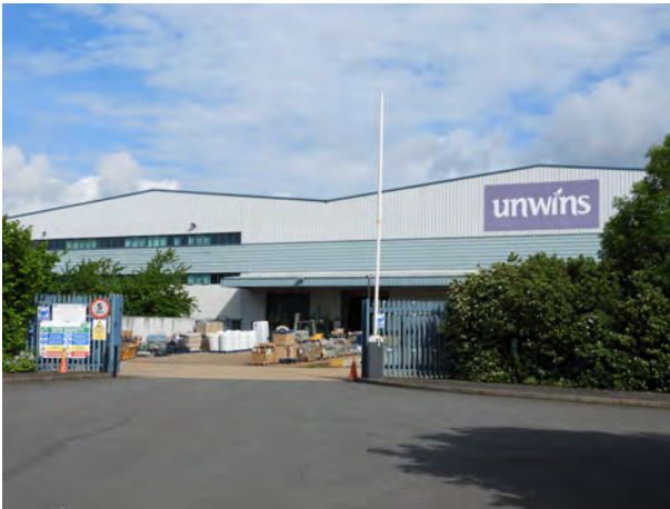
industrial unit at Alconbury Hill
