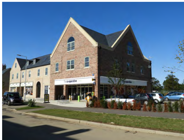
Local facilities are integral to the redevelopment of Brampton Park
