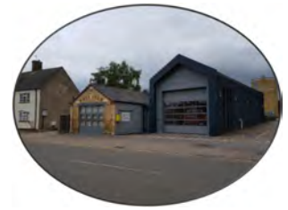
Victorian fire station building with a modern addition
