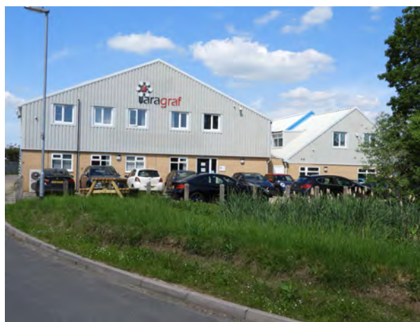
Unit within the West Newlands Industrial Estate constructed from a mixture of buff brick and cladding
