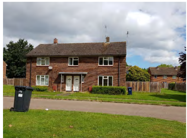
Manchester Road, former RAF Brampton. An example of lower density housing common to military sites.
