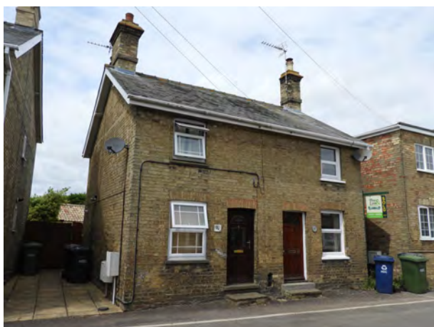
Popes Lane Victorian semi-detached homes
