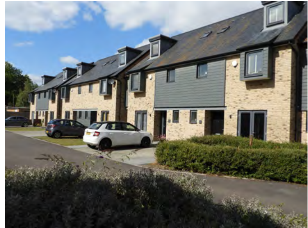
Redeveloped homes at Oldman Court
