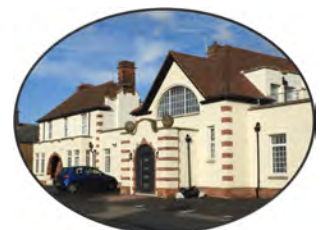
Converted Police Station on Blenheim Road
