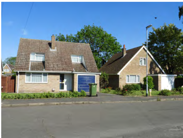
Queens Road chalet bungalows
